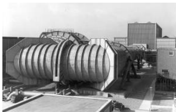
Above: the 8ft x 8ft wind tunnel at Bedford. The lamp post and cars in the foreground give an idea of the scale
